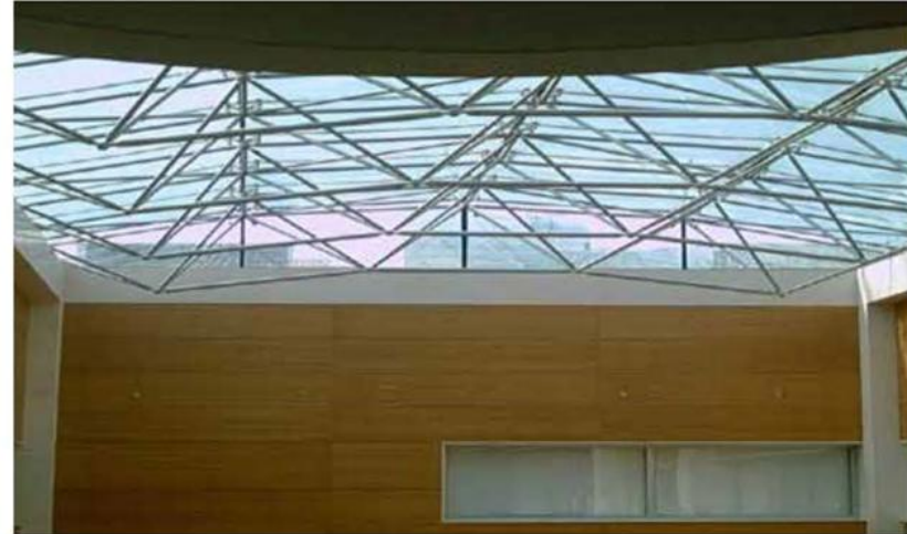
Kgl Skylight With Spiders & Space Frame
