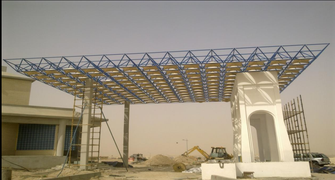
Steel Space Frame&Teflon Fabric Struc. at Ali-Al-Salem Airbase
