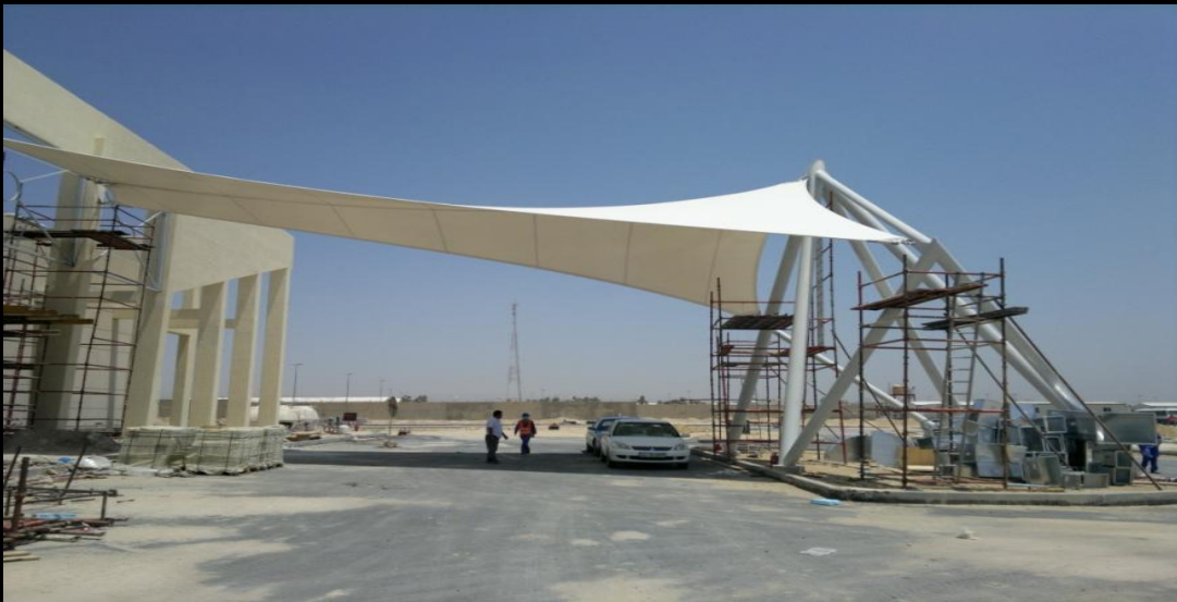
PUMPING STATION BUILDING (MINA ABDULLAH WDC -Main gate)
