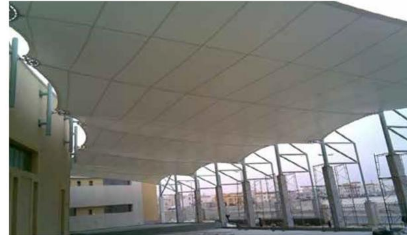
Steel and PVC structure-Entrance - Kuwait Autism Center
