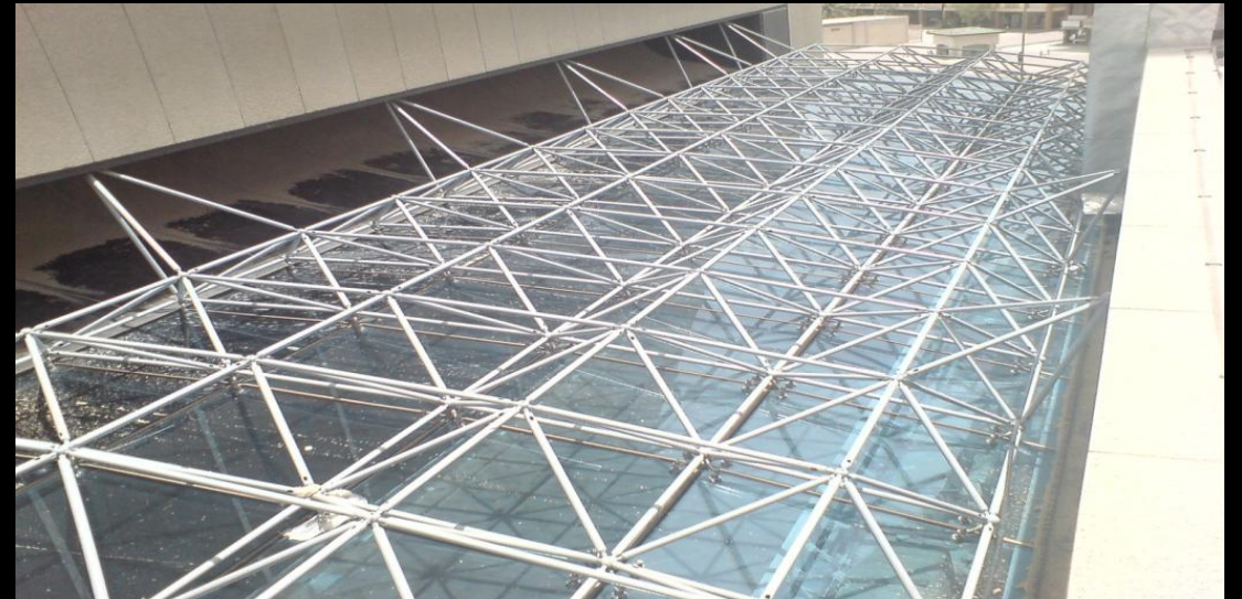
AHLI BANK VIP HALL- SPACE FRAME AND SKYLIGHT
