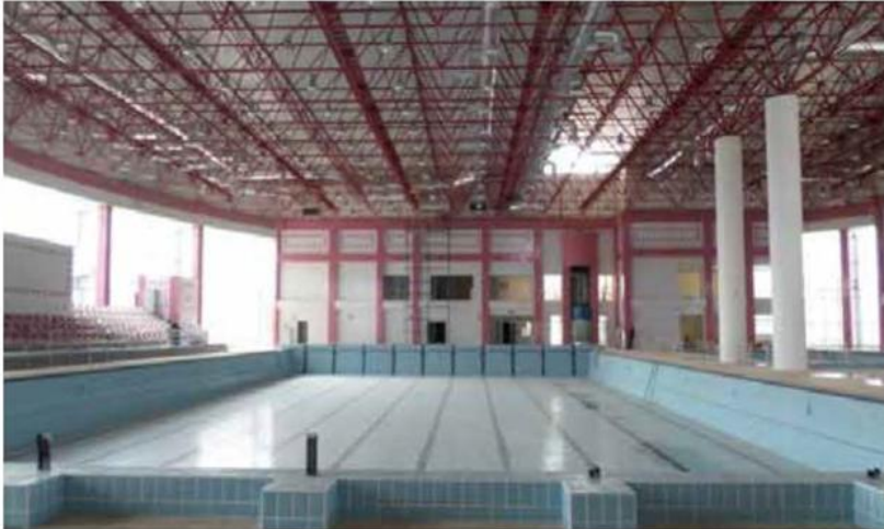
Sulaibikhat Swimming Pool- space frame and sandwich panel cladding
